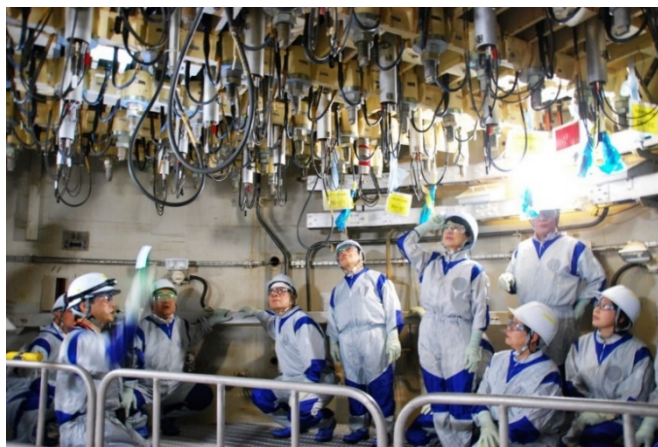
Below a pressure vessel.
