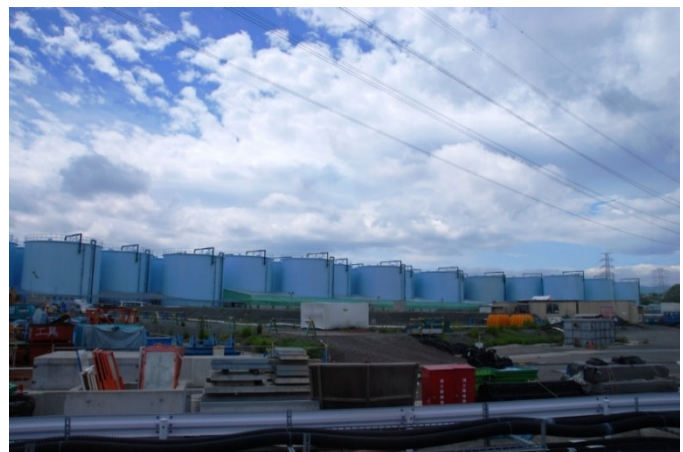
Tanks storing contaminated waters
